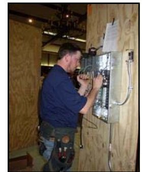
Steven Carpenter, IEC Kentucky and Southern Indiana, working on a panel.
